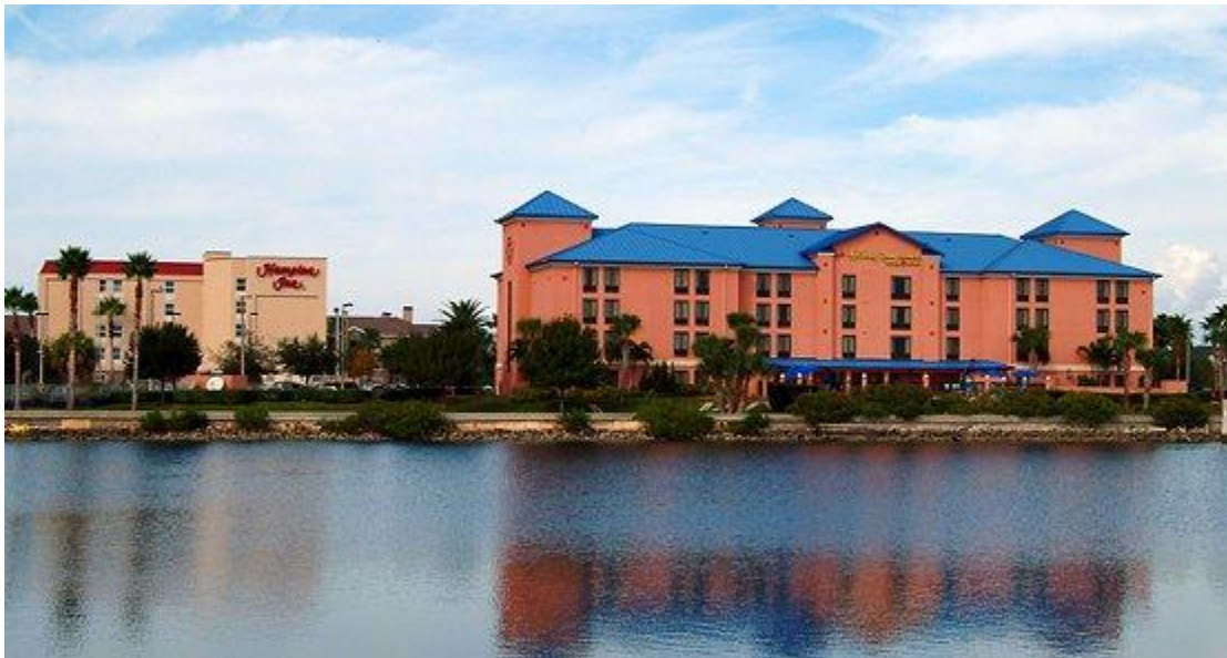
Charter One's Hampton Inn Rocky Point (left) and Holiday Inn Express & Suites Rocky Point Rocky Point Tampa, Florida
